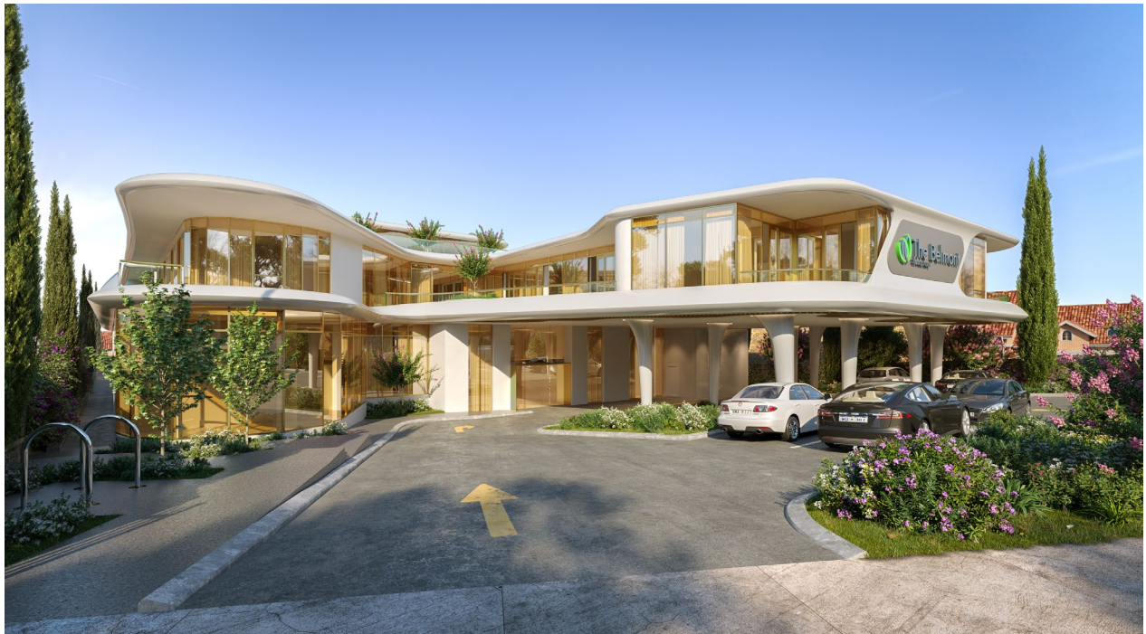
New street frontage from High Street, Belmont.
